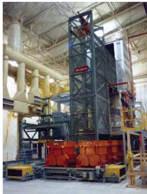
Bottom Drop Charging System
