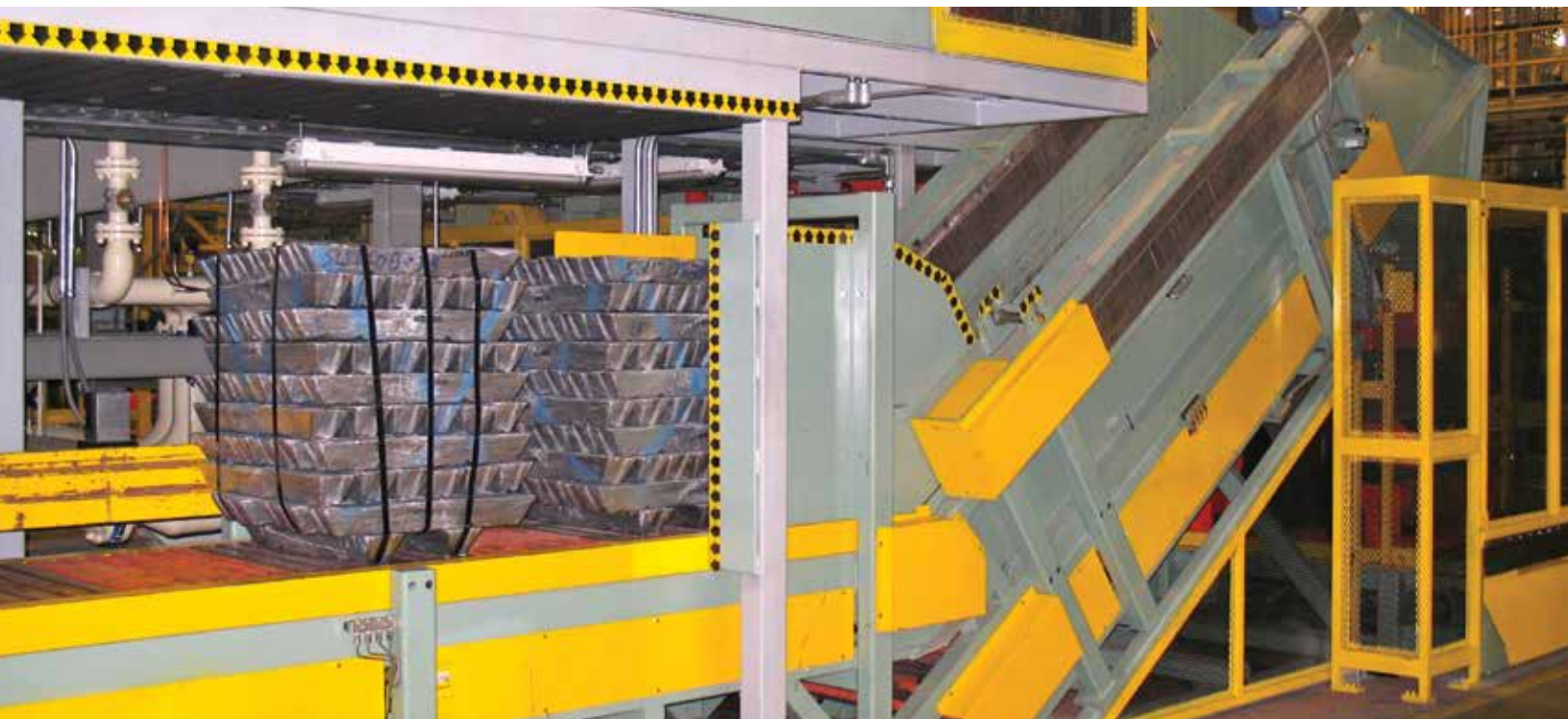
Ingot Destacking System
